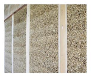
Fig. 11 Interior insulation – Master's thesis conversion of an old farmhouse, Switzerland (Photo credits: Author 2)
