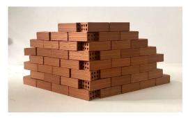
Fig. 1 Exploring different types of bonds for brick masonry structures – load-bearing solutions and aesthetic patterns
